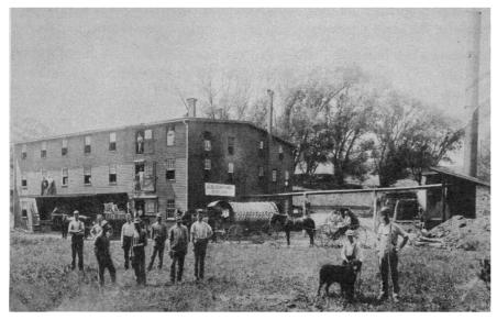
On the far right are the smokestack, boiler and steam engine building, which apparently transferred rotary-shaft power overhead to the manufacturing building on the left. [Photo from C. Milton Wright, *Our Harford Heritage: A History of Harford County, Maryland* (Glen Burnie, MD: French-Bray Printing Co., 1967), p. 142.]
